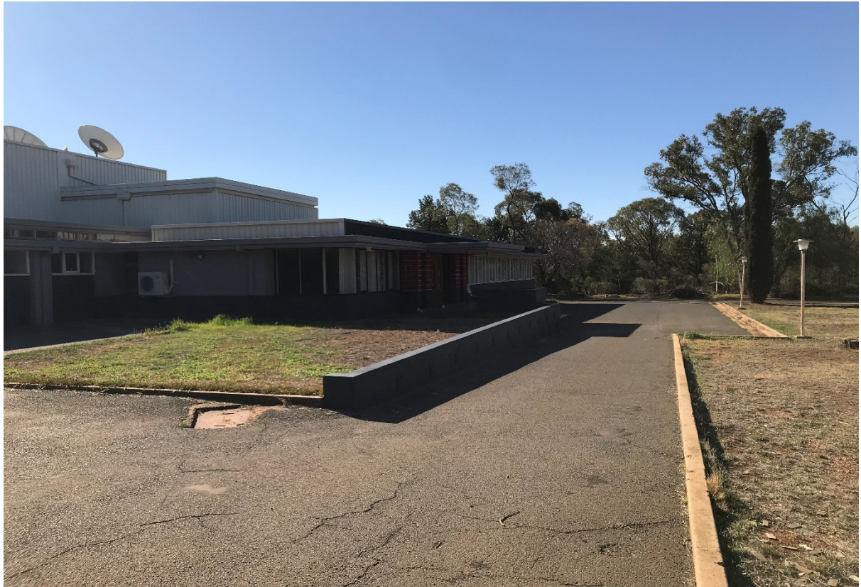
D3: Existing Building of Former MTN9 & 2RG Broadcast Centre (front elevations)
