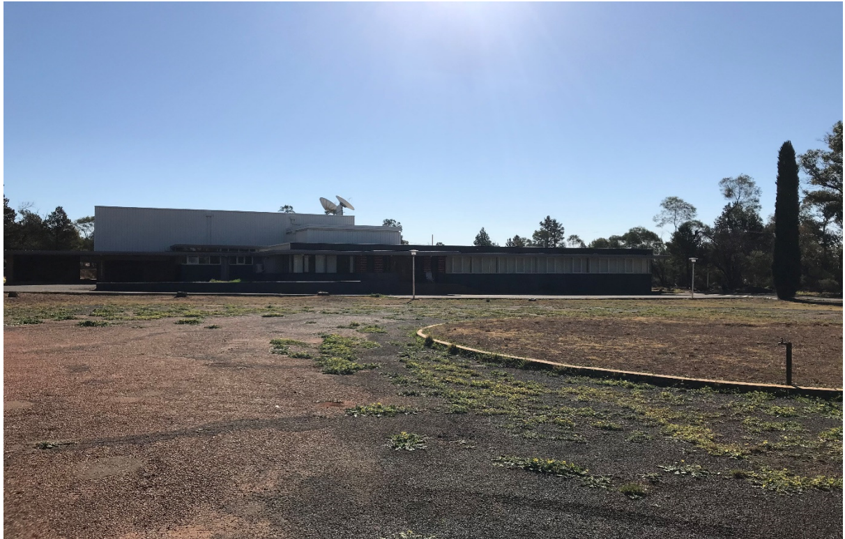
D2: Existing Building of Former MTN9 & 2RG Broadcast Centre (front elevations)
